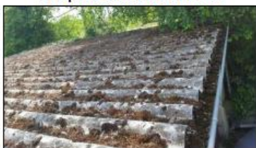
Plaques amiante ciment
