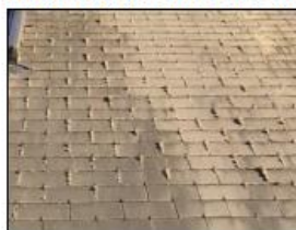
Ardoises amiante ciment
