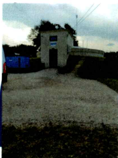
REHABILITATION RESERVOIR - LE LYCEE NONTRON
