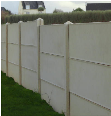
PLAQUES LISSES BETON MOULE
