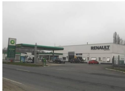
Garage - station service
