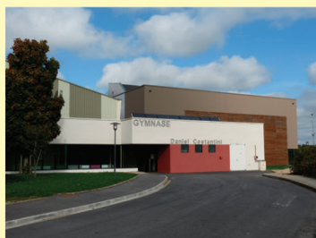
Gymnase D. Costantini
